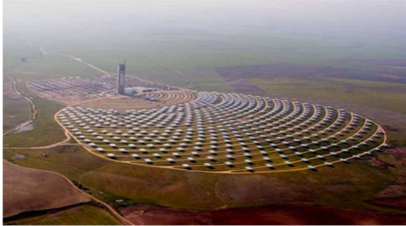
Figure 1-10 Solar power tower at Sevilla, Spain [30]
