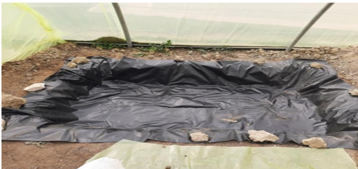
Figure 17: Second step (installation of the plastic double layer).
