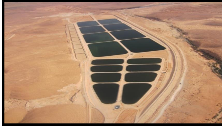
Figure 4 : la station d'épuration Kef Eddoukhan
