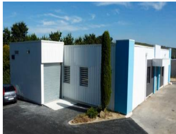
Figure I. 7 - Lightweight commercial building model incorporating PCM.
